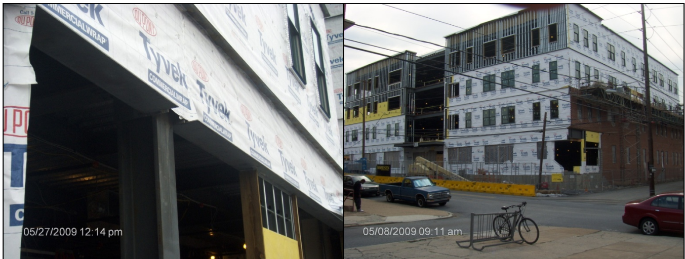
Figure 30 – Masonry Façade Steel Support Angles
