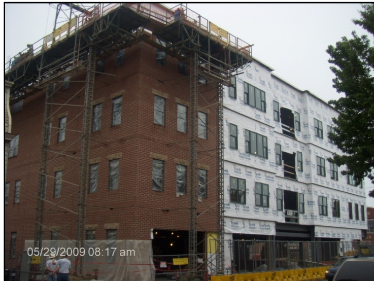
Figure 10 –Installation of the Exterior Wall System
